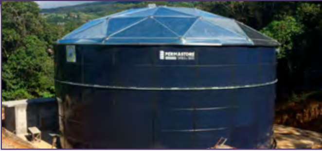
1: Geodesic Dome Roof – Costa Rica
