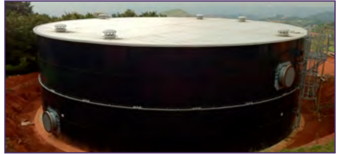
4: Trough Deck Roof – Drinking Water
