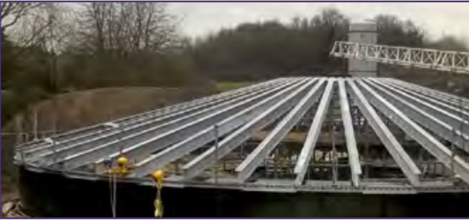
3: External Beam Roof – Anaerobic Digestion & Biogas
